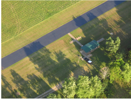
Aerial view of runway after sealing completed (photo thanks to R. Dombek)
